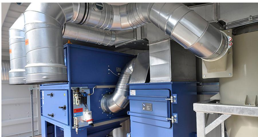
The "ZPF" suction and filter system is able to extract and clean large volumes of contaminated air: Two sets of pipework – one for welding fumes and the other for dust from grinding work – extract the contaminated air and guide it via the pre-separators to the filter unit.
